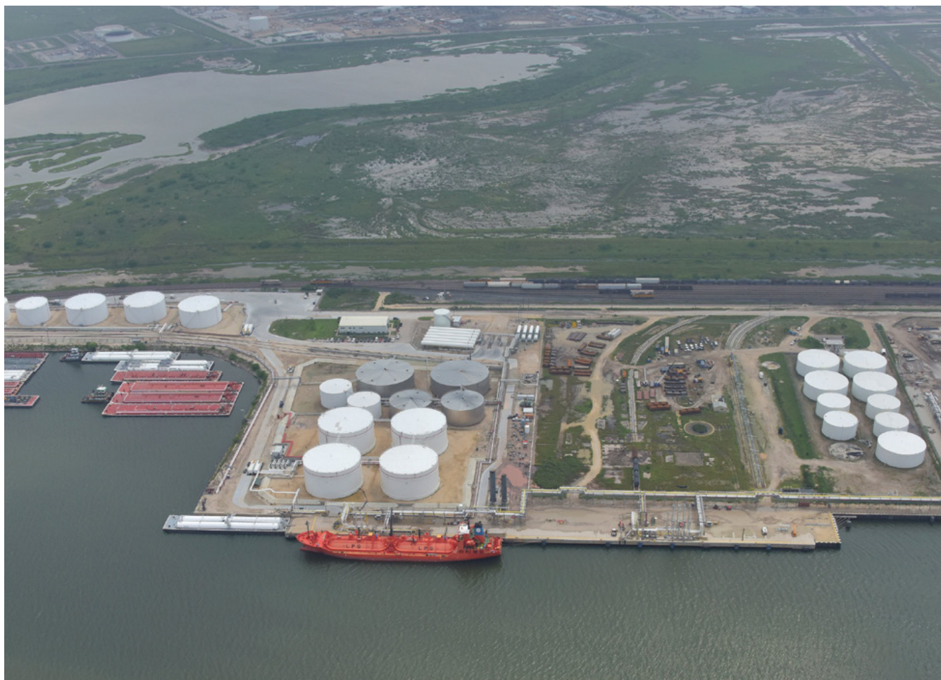
Corpus Christi oil storage facility, Texas, US.
